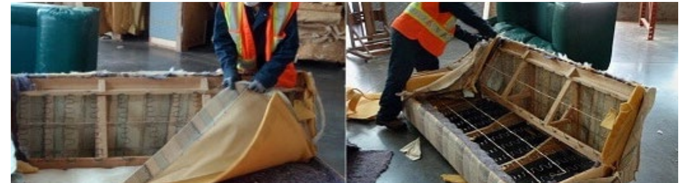
Wood frame and polyurethane foam cushion
