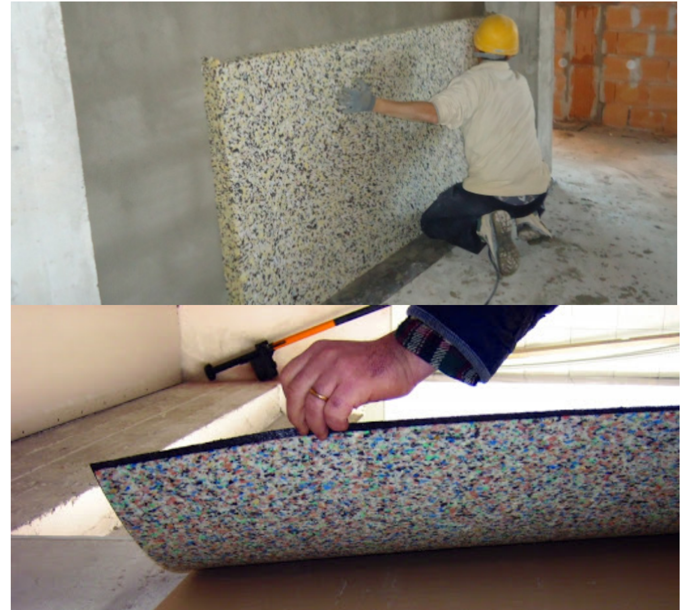
Recycled polyurethane insulation boards are easy to install, mouldable and adaptable to different building shapes.
